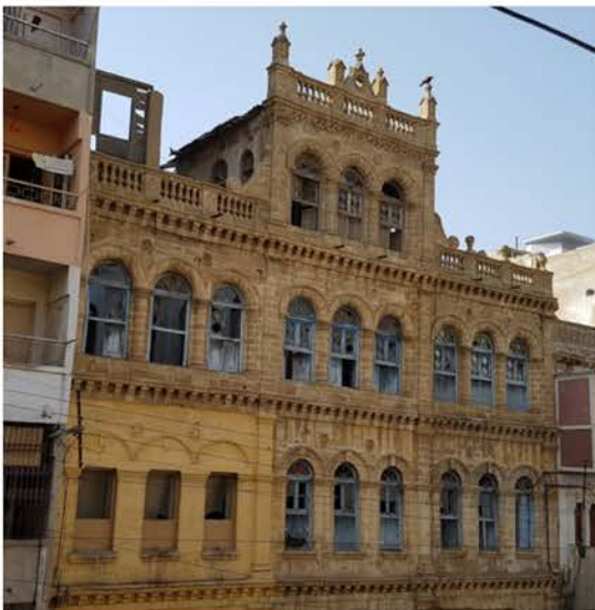
Kanji Building Before demolition
