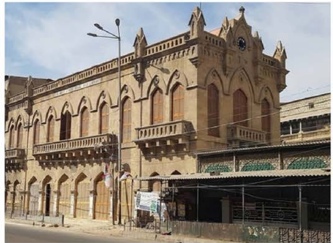
Max Denso Hall and Library after conservation
