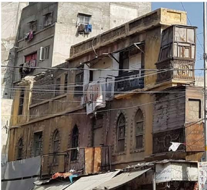
Flat Iron Building before conservation
