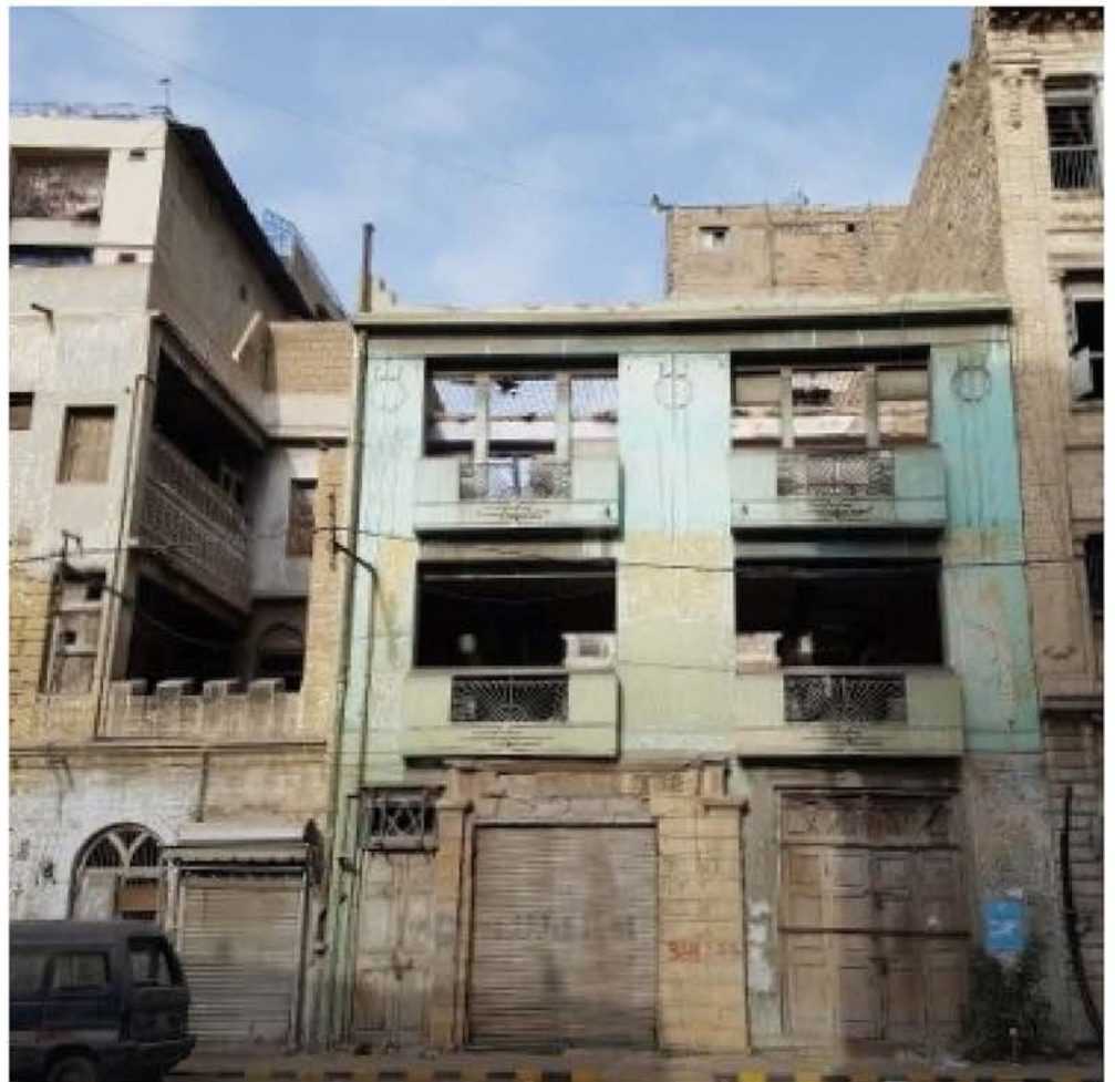
This building is shown during the walk to show the process of demolition of an art deco style building.
