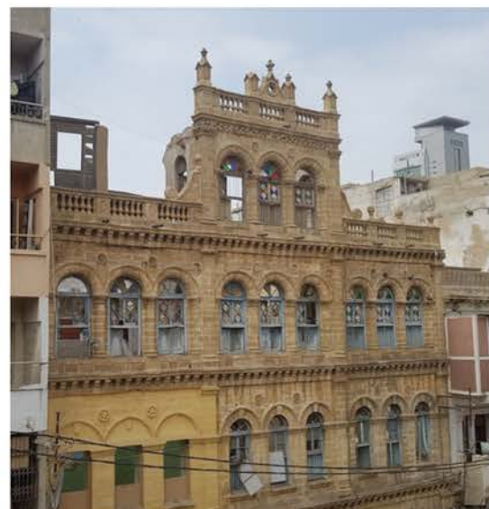
Kanji Building after demolition, now a free standing facade
